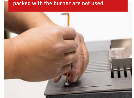
3. Unpack the burner from the packaging and mount it on top the base frame with the four stainless steel screws M5.
